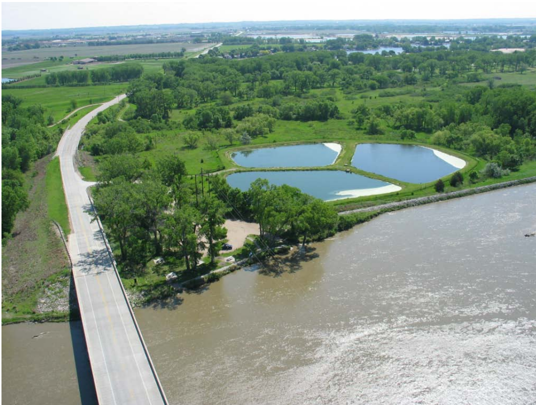
Photo 3: Highway 64 Bridge, Platte River Landing near center, and treatment ponds.
