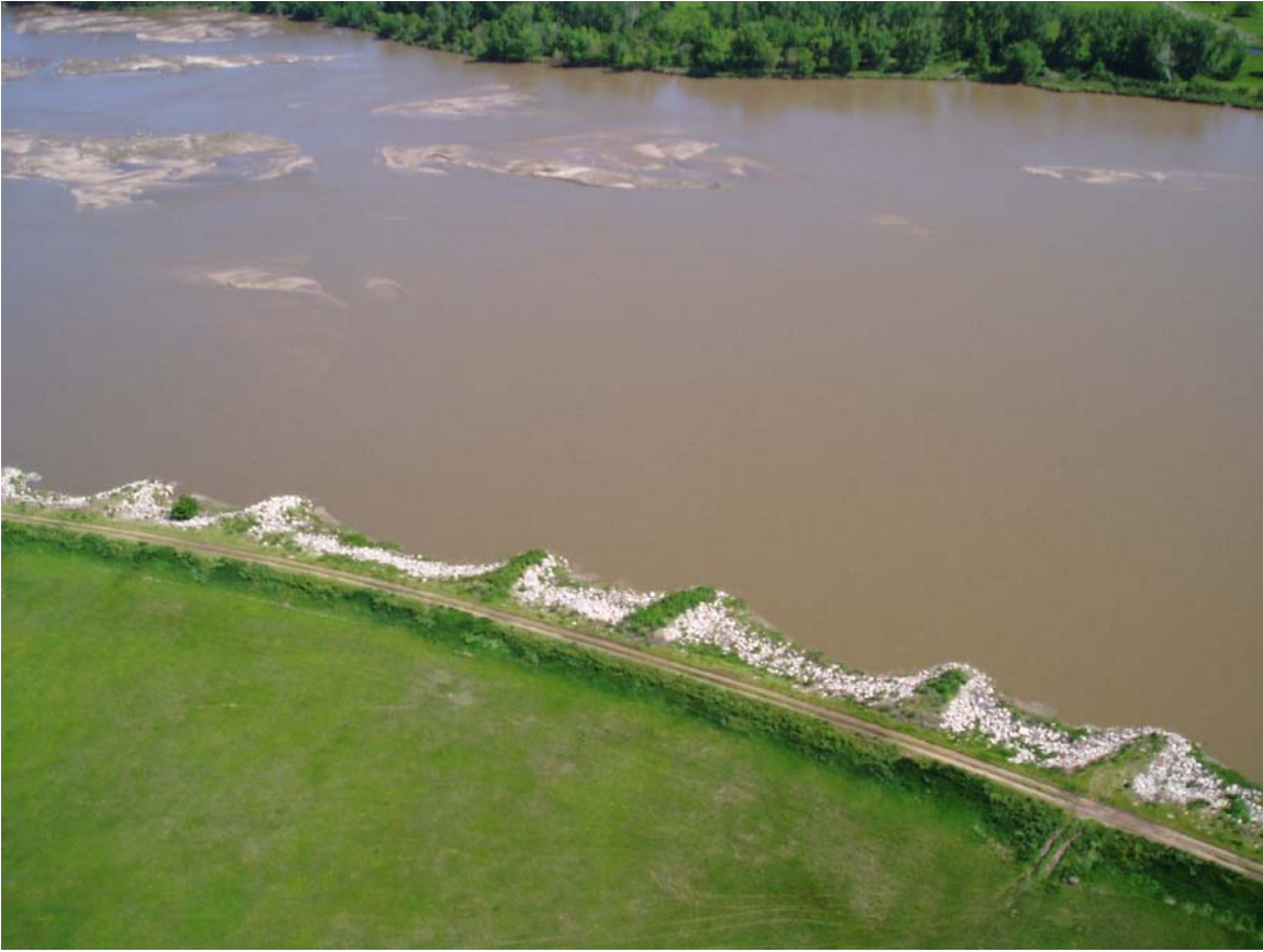
Photo 2: Typical levee and bank stabilization along the Platte River.
